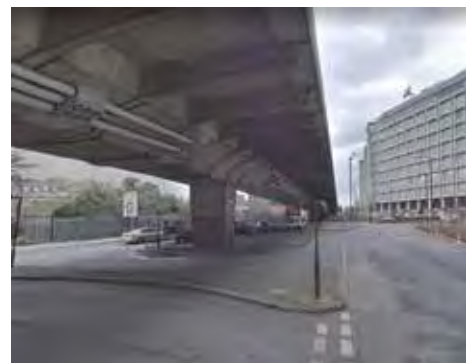
A4 Flyover looking west
