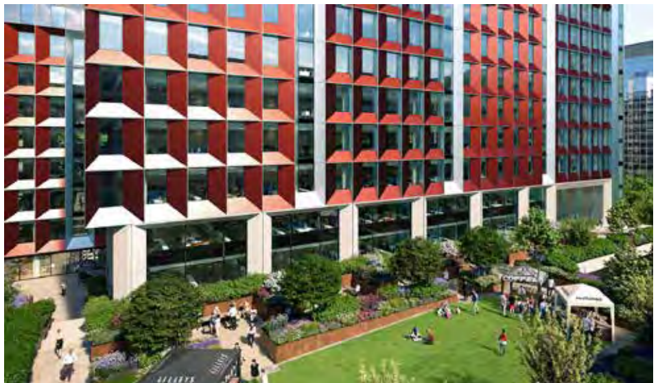
Podium Gardens behind 245 Hammersmith Road
