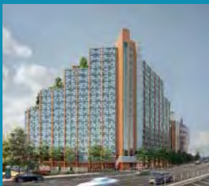
161 Talgarth Road - Under Construction
